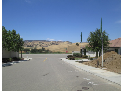
Looking north along Golf Canyon Drive – Villa Vista Subdivision
