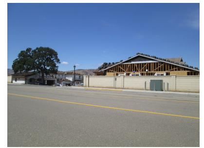
Villa Vista Homes under construction along Fairway Drive
